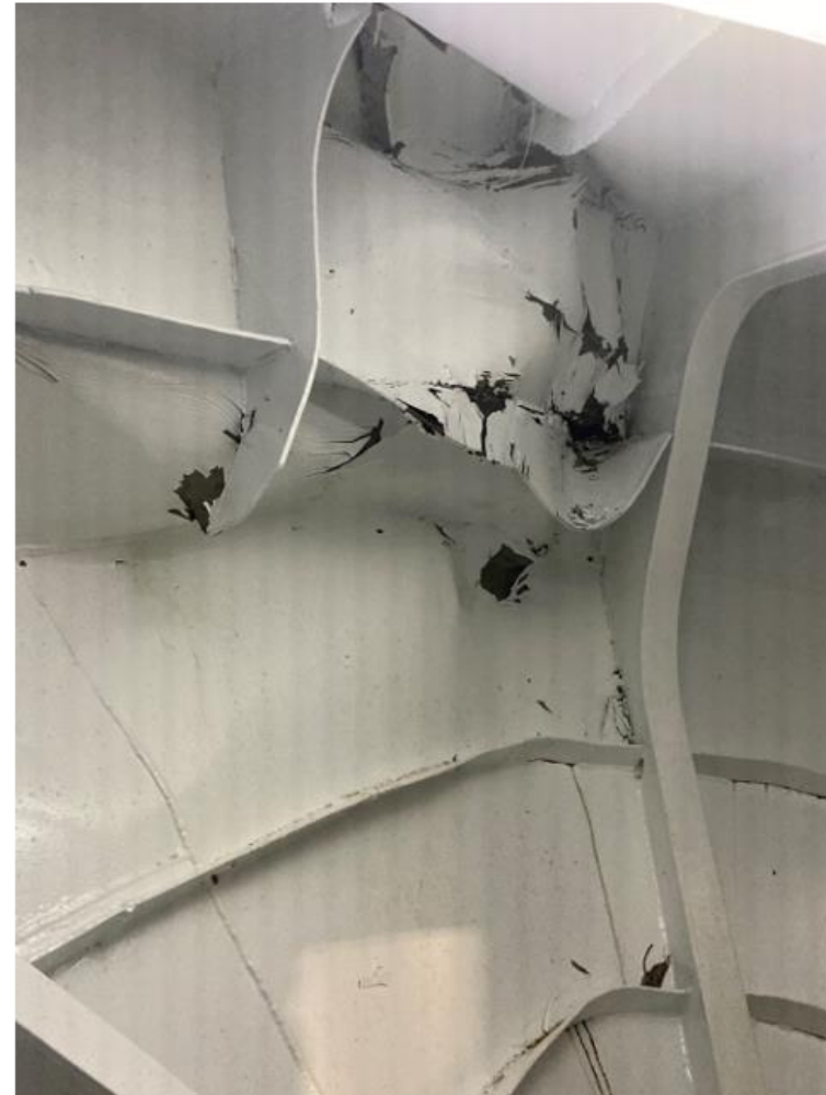
Picture of Fore Peak showing damage to shell plating, Frames and stingers. Stem Frame on right of photo. Port 01 (Intermediate) Frame on centre left
